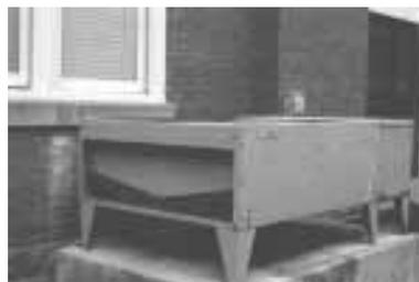
**Figure 29.** Air-cooled condenser.
