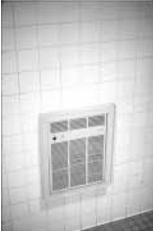
**Figure 17.** Built-in electric resistance heater.
