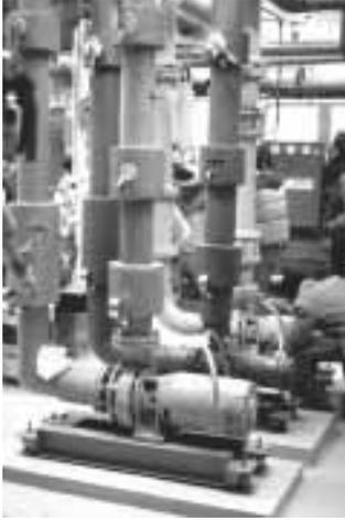
**Figure 35.** Centrifugal pumps.
